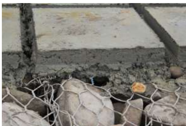
Figure 1 Well-constructed concrete abrasion resistance pad
