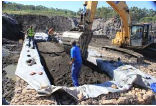
Figure 5 A stage in the construction of a compacted granular fill for a weir
