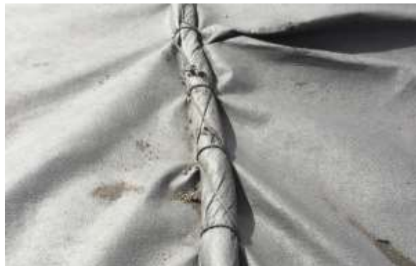
Figure 6 The joining of geotextile sheets by rolling and stitching with suitable wire
